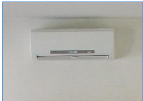
Figure 9: Wall Mounted Indoor Unit
