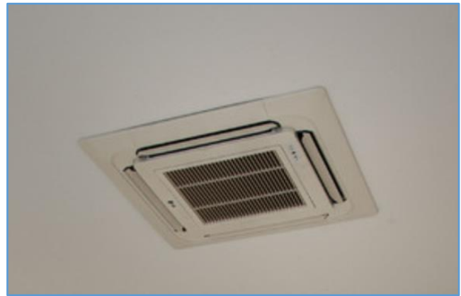
Figure 11: Ceiling-mounted Indoor unit
